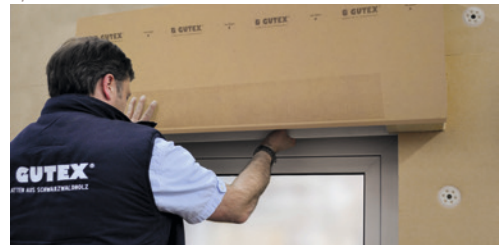
Installing the housing after insulation board installation
