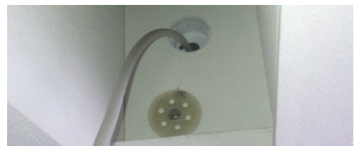
Fastening on the ends with GUTEX Thermowall® Holzschrauben (wood screws)
