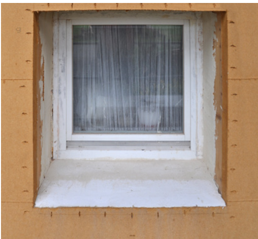
Trowel-smoothed surfaces with GUTEX Durio facade installed over an old facade
