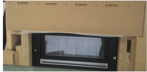
Installing the housing during installation of the insulation boards
