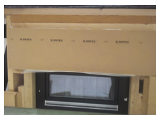
Installing the housing during installation of the insulation boards
