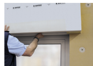
Installing the housing after installation of the insulation boards
