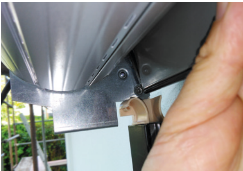
Feeding the sunshade into the tracks
