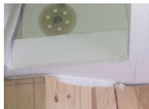
Fastening on the ends with GUTEX Thermowall® Holzschrauben (wood screws)
